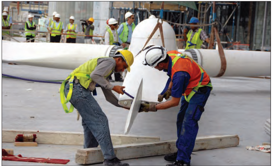
Sangill ... happy with the turbine tests. RIGHT: Engineers check the blade tips which can act as a mechanical fail-safe brake in case of an emergency.
