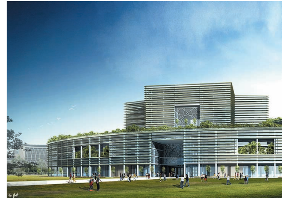
IMAGE: The Putrajaya Precinct 2 - 2C5 project in Malaysia is targeting a LEED rating of Silver.
